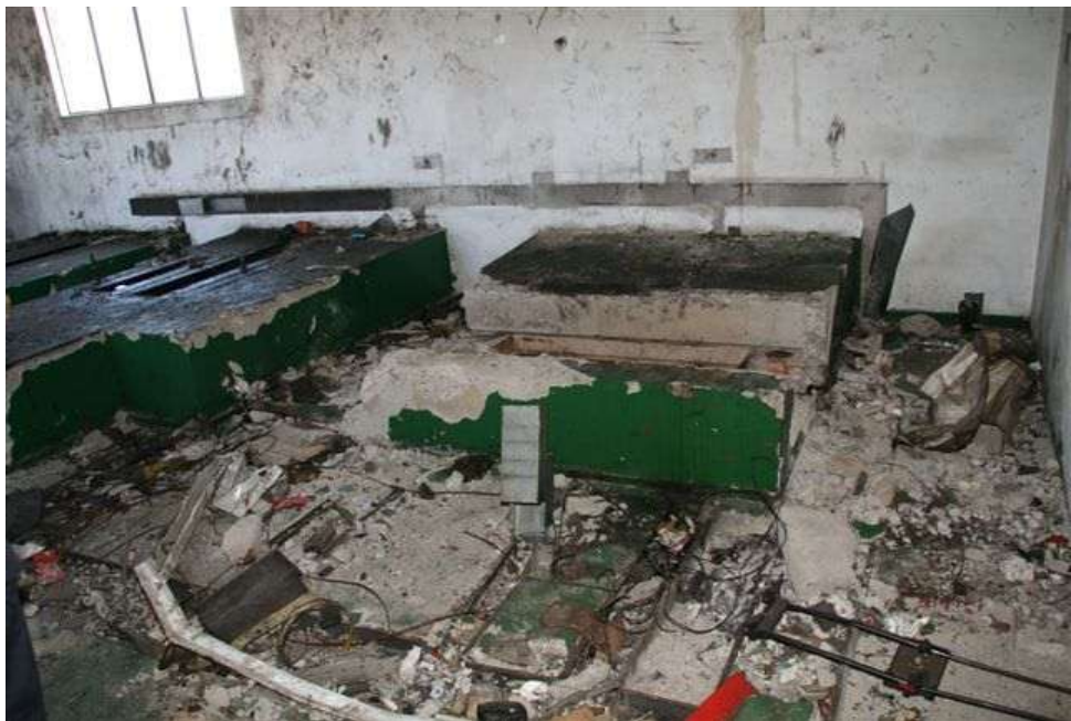
All items removed from the lift room such as the motors, switch gear and electrical distribution boards
