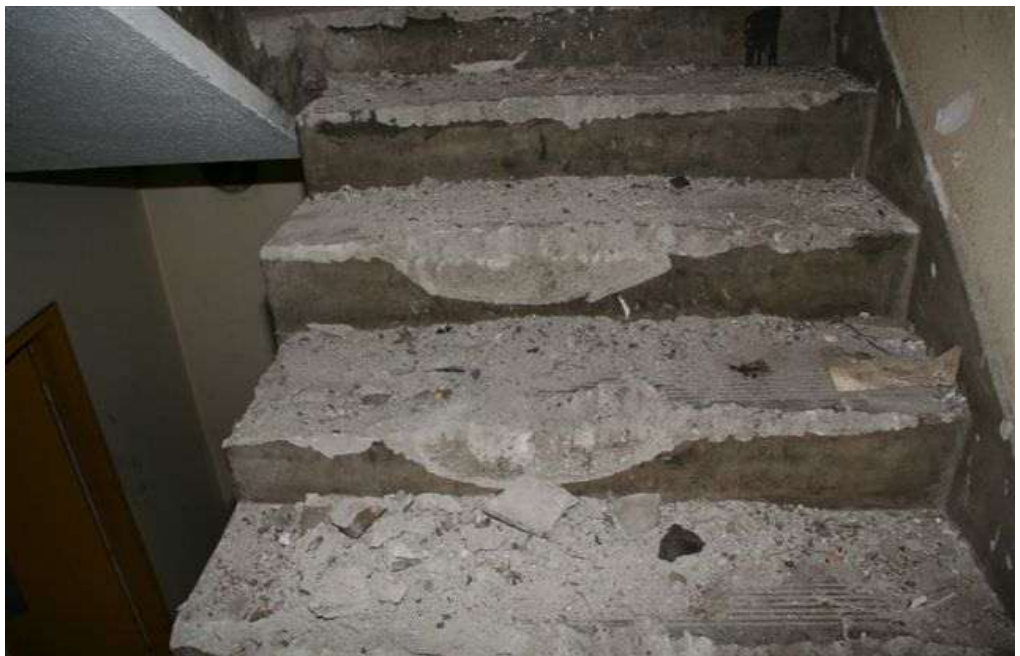
Stairs that have been damaged by the vagrants when they removed the lift motors and lifting mechanisms and dragged them down the stairs.
